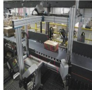
Multiple integrated distribution and fulfillment systems (including laser-based identification and dimensioning technologies) communicate in a warehouse to identify and route items and parcels through the facility and out to a customer.
